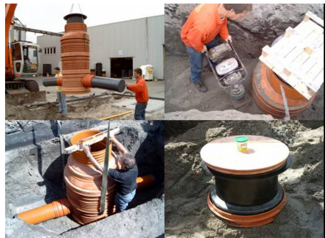
Figure 5: Impression of burying the 800 and 1000 manholes
